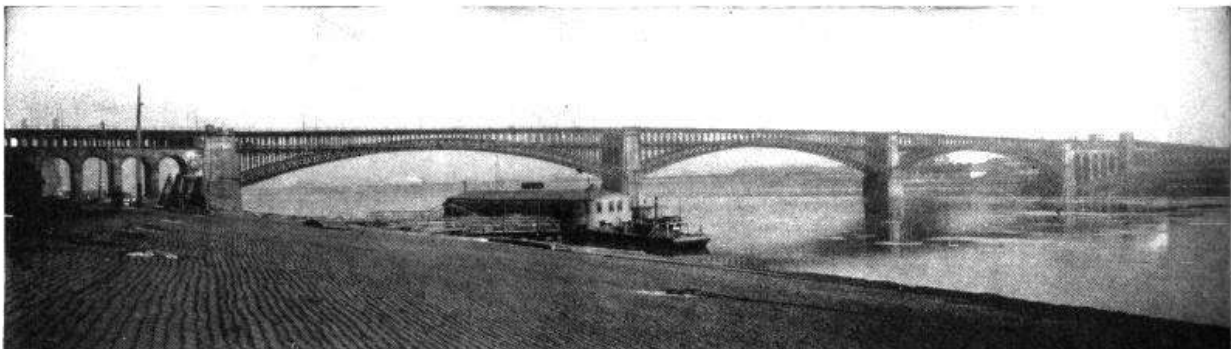
EADS BRIDGE, ST. LOUIS
